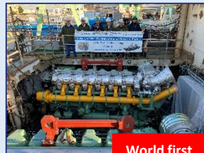
February 2024 Main Engine installed to A-Tug
