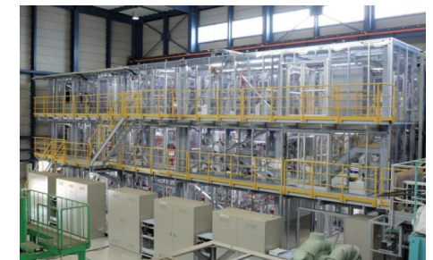
Hydrogen production test apparatus of IS process
