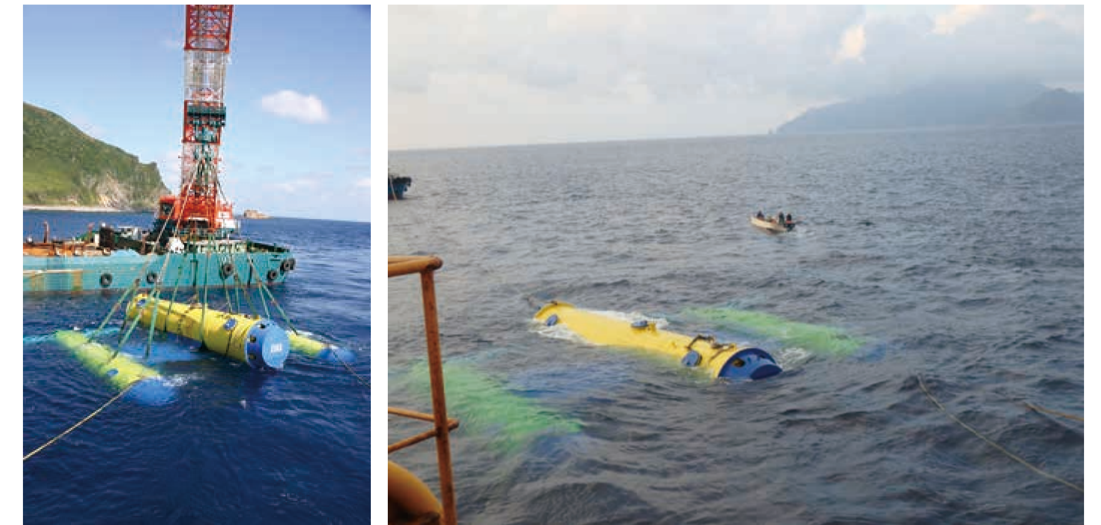
Subsea Floating type ocean current power generation system; installation image
